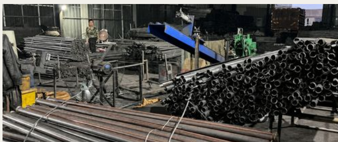
Steel Tube Material Staging Area WORKSHOP
